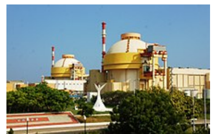
The Kudankulam Nuclear Power Plant
