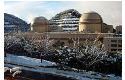
The Ōi Nuclear Power Plant
