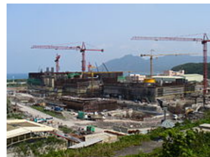
The Lungmen Nuclear Power Plant under construction (now halted)
