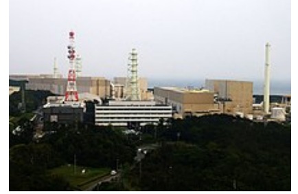
The Hamaoka Nuclear Power Plant
