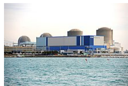
The Kori Nuclear Power Plant
