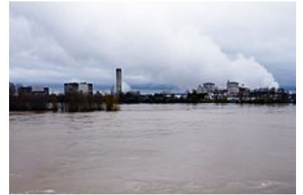
The Chinon Nuclear Power Plant
